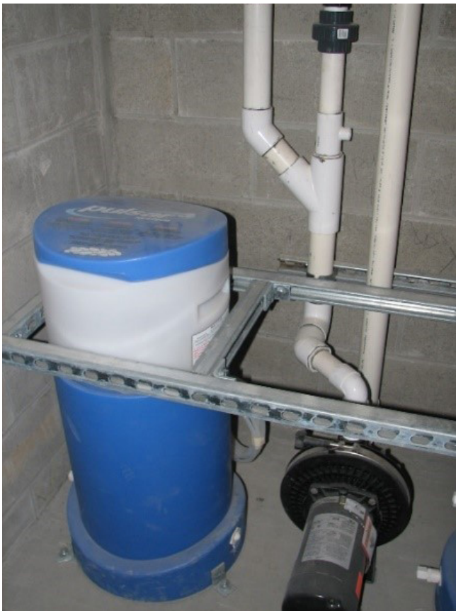
Figure 8: Proper Calcium Hypochlorite Storage
